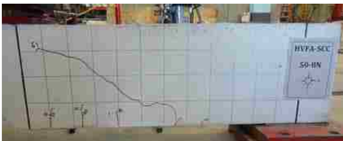
Figure B-5. Cracking Shear in Specimen 50-8N
