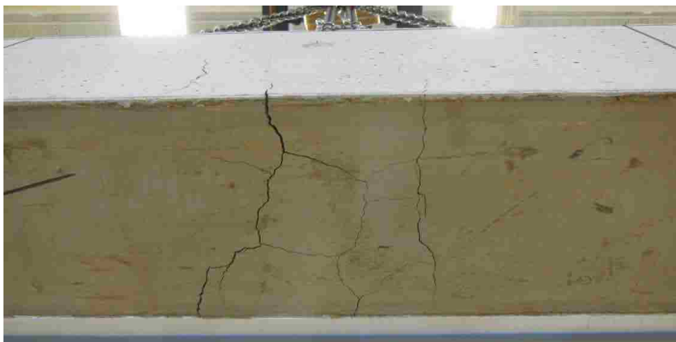
Figure D-6. Crack Pattern of Specimen BWC-50 (Bottom View)
