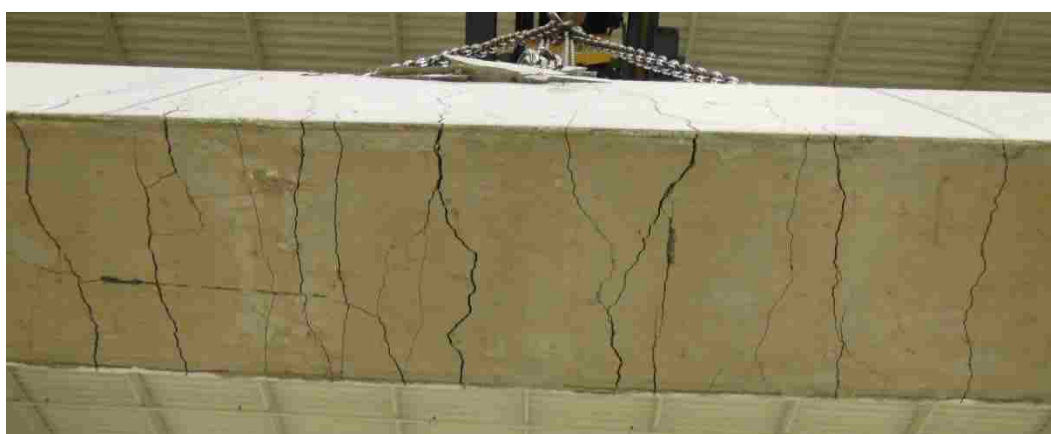
Figure D-2. Crack Pattern of Specimen REF-50 (Bottom View)
