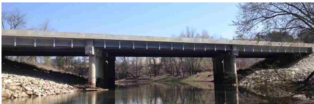
Figure 4. Bridge A7957 during the summer
