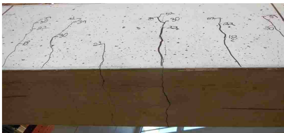
Figure D-22. Crack Pattern of Specimen BWC-70 (Bottom View)
