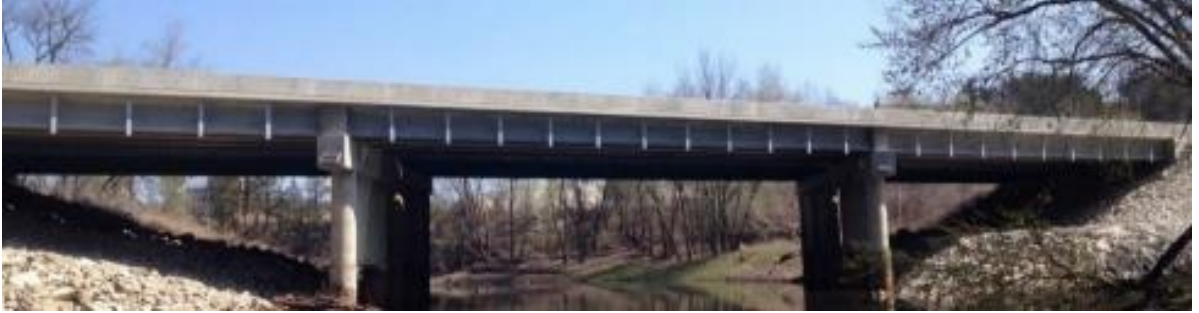
Figure 2. Bridge A7957 during the summer.
