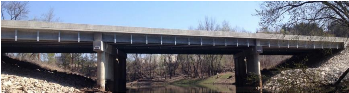
Figure 1.9. Bridge A7957 Side View
